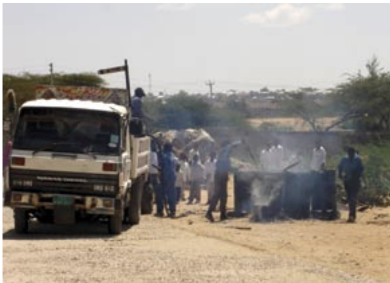
Road building provided by Hargeysa's municipal authorities, March 2006
